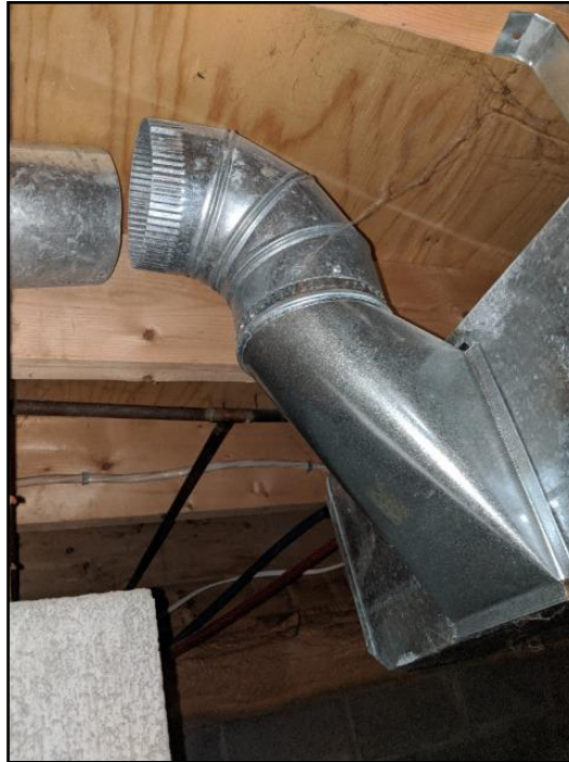
11. Disconnected ducts
