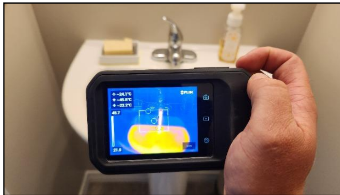
20. Water hot at time of inspection
